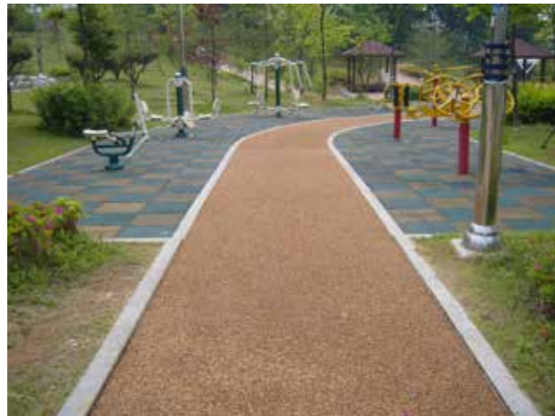
Fig. 3.20: EPDM tiles used for outdoor-gym area, compacted wood chips for jogging track. (Neung-in Park, Namdong-gu, Incheon)
