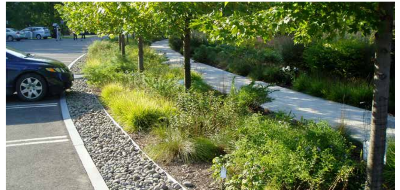
Fig. 3.46: Bioswale along the parking bay, in Tompkins county, New York. (Cornell Plantations Bioswale, Green Infrastructure around Tompkins county, Stormwater coalition of Tompkins County, New York, USA)
