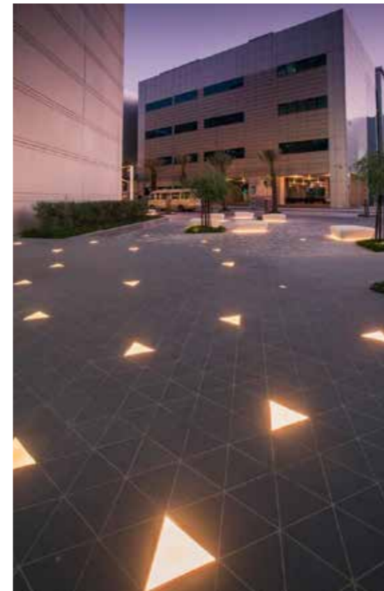
Fig. 3.35: Luminaires integrated seamlessly into the similar shaped pavement, Khalifa University Extension, Abu Dhabi. (Custom made LED luminaires: Exterior Lighting Product of the year award, Khalifa university extension, Abu Dhabi, 2017)
