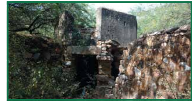
Fig 2.8: Lack of preservation of structures of historic importance. (DUAC)
