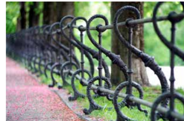
Fig. 3.42: Ornamental metal fence. (Park metal fence, uploaded by YandeG, 2015)
