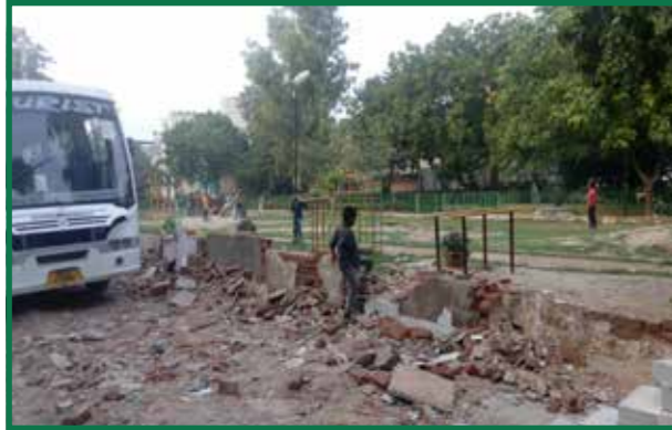
Fig 2.11: Dilapidated boundary walls and fencing without gates and defined approach. (DUAC)
